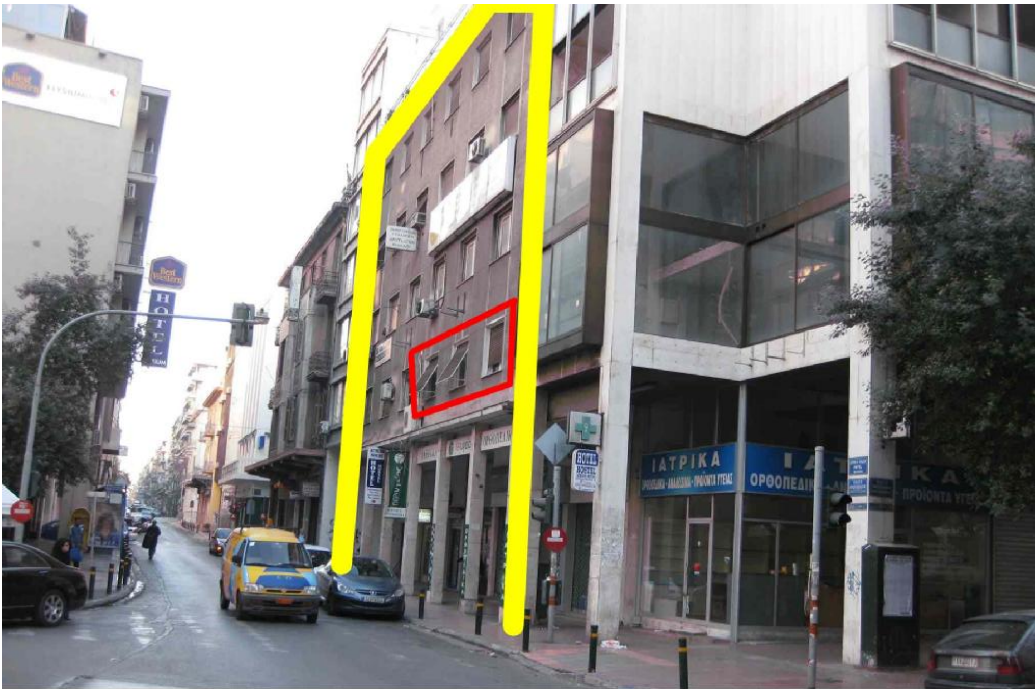
Building in Yellow, Offices for Sale in Red. Photo taken with view towards Patissia
